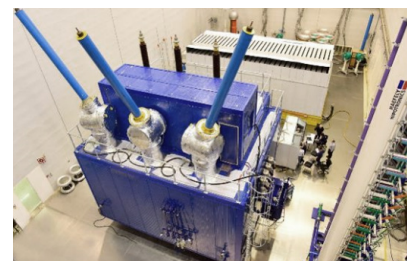
Transformer 300 MVA three-phase Autotransformer
