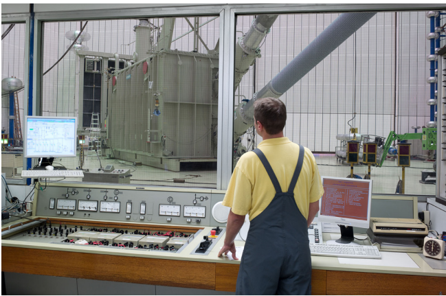
For testing, the transformer is completely set up and connected
