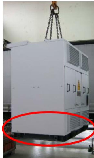
Image 5-23: Opening of the enclosure roof to attach the crane hooks to the transformer
