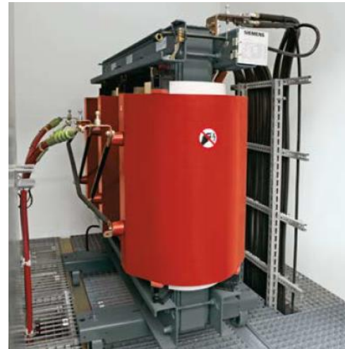
Image 6-2: Example of cable routine
