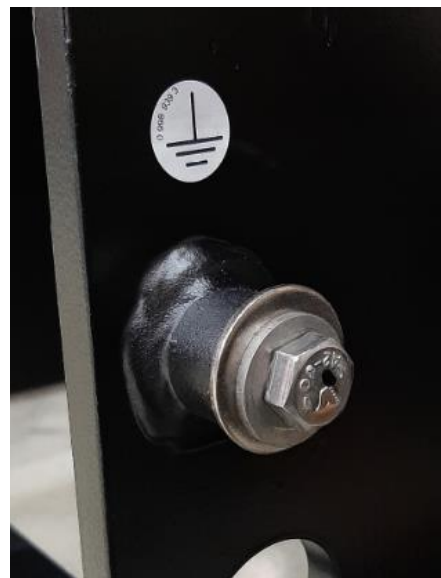
Image 6-9: Bolt for grounding connection
