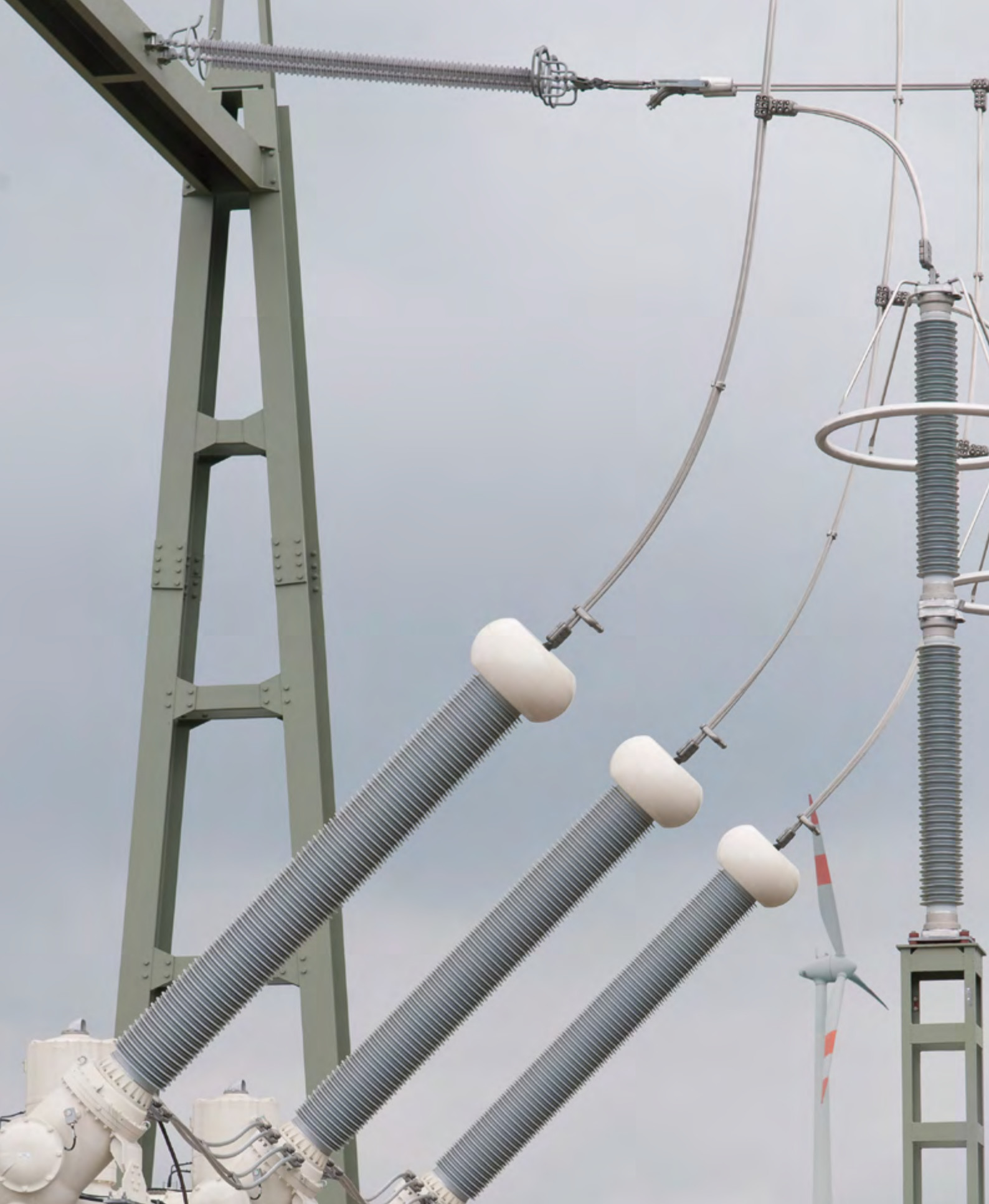
Substation Bidingen 400 kV Protection of switchgear solution with 3EQ4
