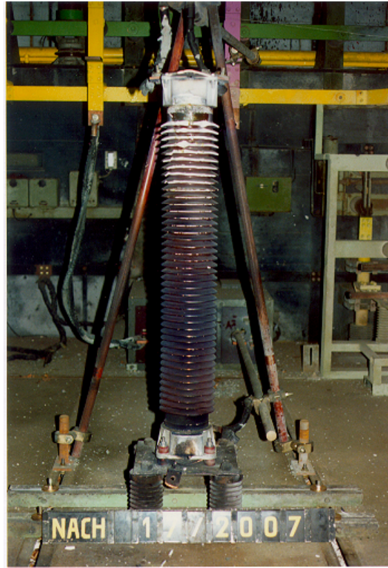
Figure 27: Porcelain-housed arrester after a test at rated short-circuit current (63 kA, 200 ms). Apart from a few broken sheds, the housing has remained intact.
