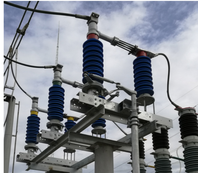
Fig. 08 Side-break disconnecter
