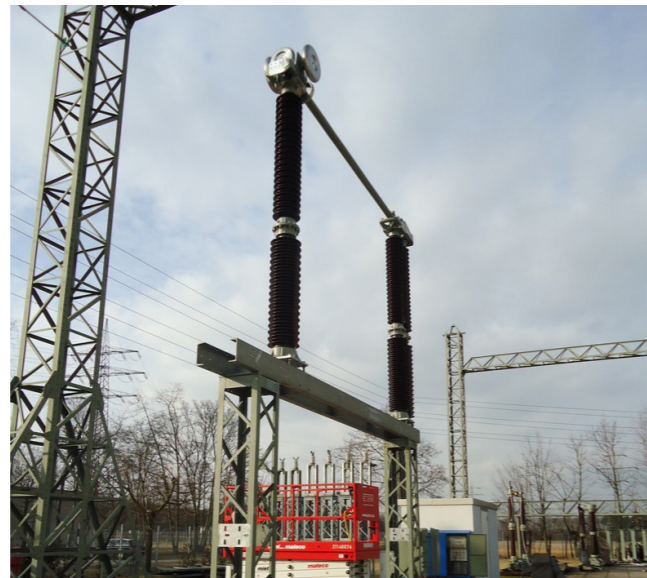
Fig. 05 Vertical-break disconnecter
