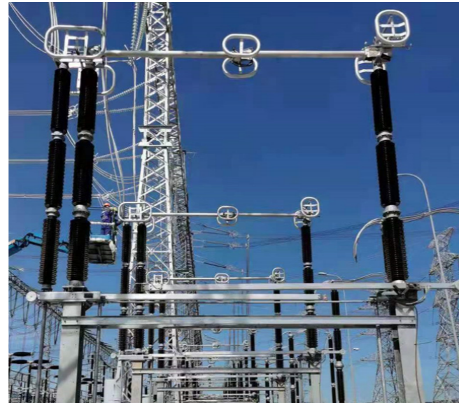
Fig. 06 Knee-type disconnecter
