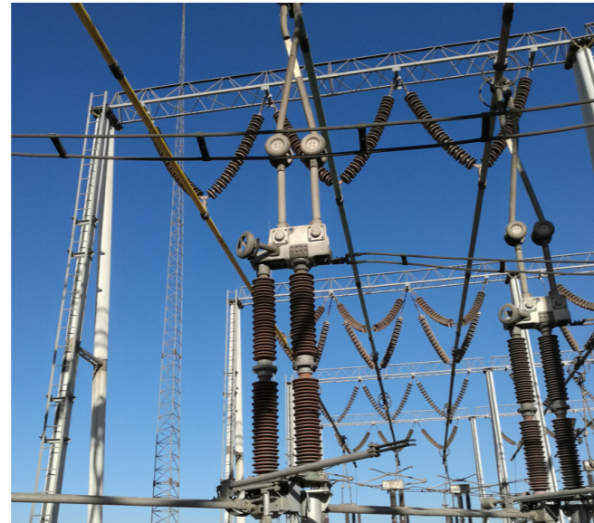
Fig. 04 Pantograph disconnector
