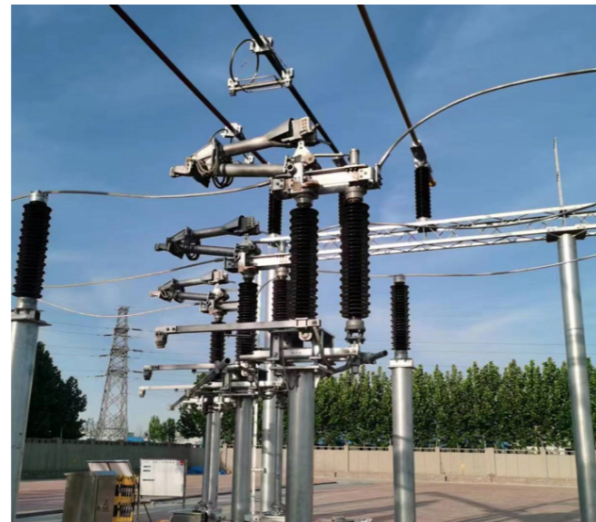
Fig. 09 Semi-pantograph disconnecter
