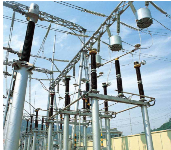
Fig. 03 Double-side break disconnecter
