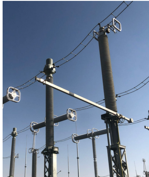
Fig. 01 free-standing earthing switch
