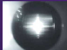
Closed earthing switch contact
