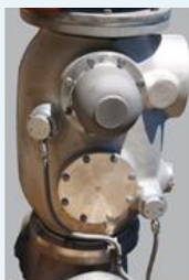
Fixed mounted cameras on the disconnecter and earthing switch module
